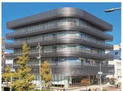
New Nakayama Memorial Hall (completed on September 15, 2021) Area of grounds: approx. 1,401 m<sup>2</sup> Floor area: approx. 5,712 m<sup>2</sup> Structure: 1 underground level, 5 floors above ground, equipped with isolation system
