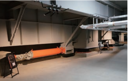
Seismic isolation equipment in Planet Saitama
