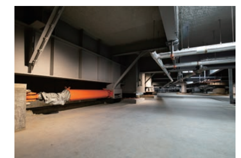
Building's seismic isolation structure allows for shipping even during disasters see p.51
