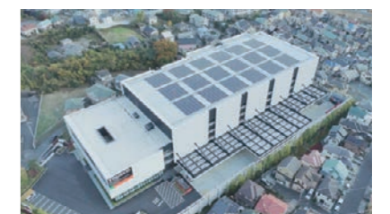
Solar power generation equipment at Planet South Kanto (Power Generation Capacity: 300 kW) (Number of Solar Panels: 1,190)
