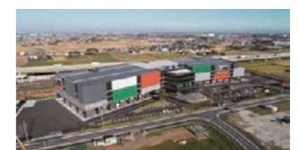
Owning our own buildings allows us to strengthen functionality (Planet Saitama Distribution Center)
