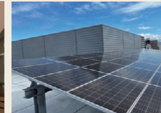
19 kW of solar power generation
