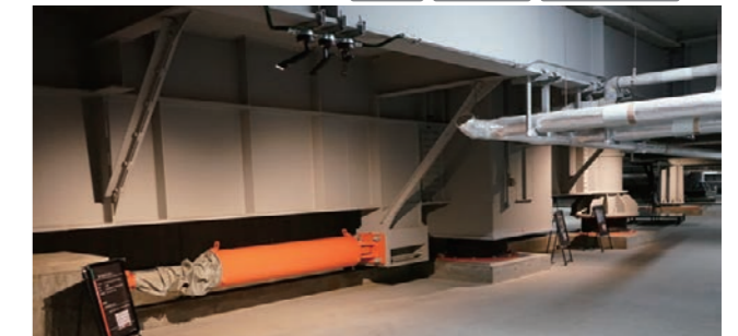
Seismic isolation equipment in Planet Saitama
