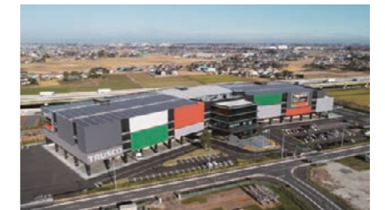
Planet Saitama Distribution Center
