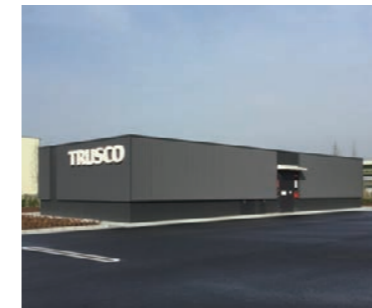
Hazardous material warehouse at Planet Saitama (approx. 284 m)
