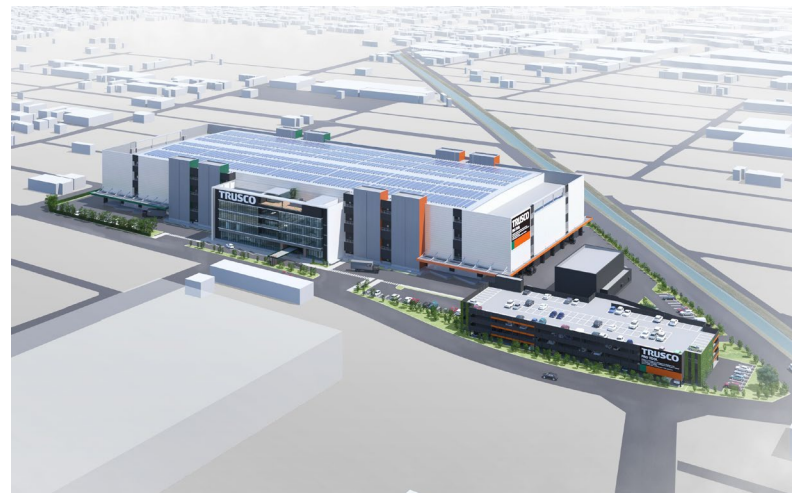
Image of a completed Planet Aichi ⇒
