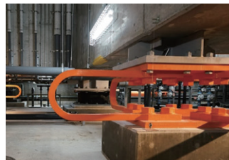
Seismic isolation equipment at Tokyo Head Office
