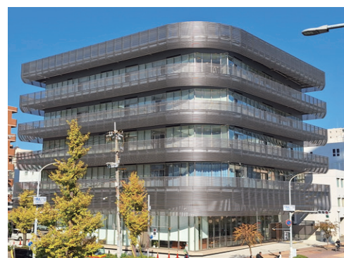
New Nakayama Memorial Hall (completed on September 15, 2021) Area of grounds: approx. 1,401 m 2 Floor area: approx. 5,712 m 2 Structure: 1 underground level, 5 floors above ground, equipped with isolation system
