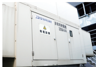
350Kva emergency power generator
