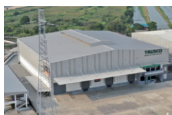
TRUSCO Nakayama Thailand Site area: 10,942 m 2 Total floor area: 4,731 m 2
