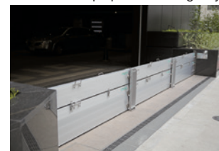
Water gates to prevent flooding, Tokyo Head Office
