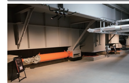
Seismic isolation equipment in Planet Saitama
