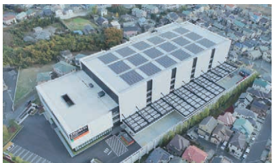
Solar power generation equipment at Planet South Kanto (Power Generation Capacity: 300 kW) (Number of Solar Panels: 1,190)
